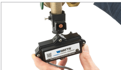
5. Press the activation module onto the sensor.
