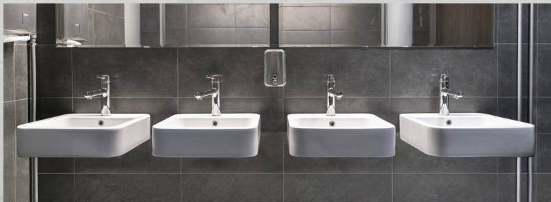
Install multiple sinks at once
